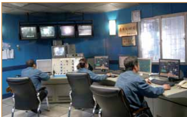
ISA Smelter Control Room at Kunming, China
